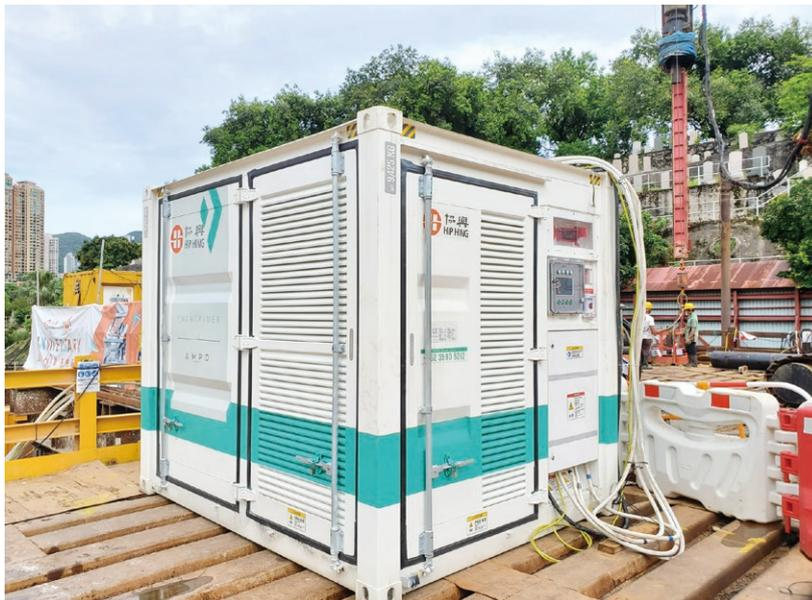
The BESS replaces the conventional diesel generators
